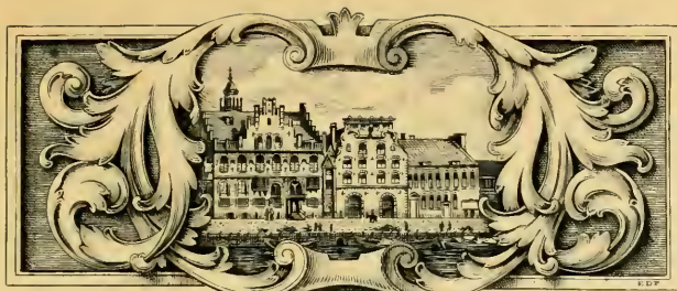
WEST INDIA COMPANY'S HOUSE AMSTERDAM - 1673
